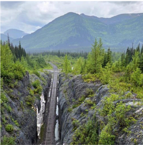
Photo: Backcountry Bandit - Sukunka Tunnels
